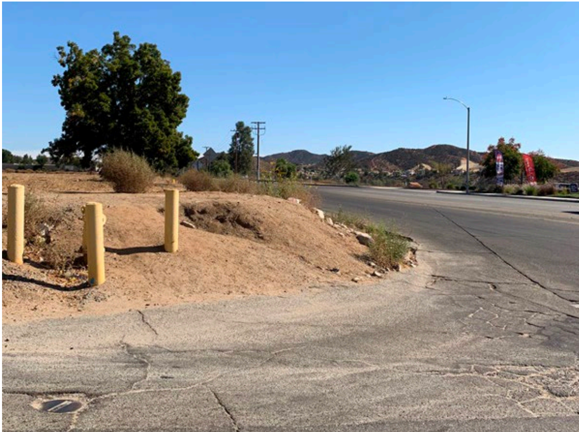
Figure 3.12: Sight Distance Blocked by Mud Mound for Vehicles Turning out of Cherry Street
