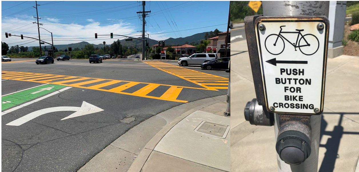
Figure 3.28: Push Button for Bike Crossing at the Intersection of Palomar Street and Clinton Keith Road
