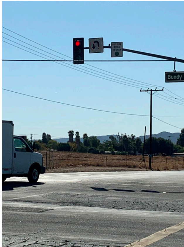
Figure 3.6: Faded “No U-turn” Sign of Southbound Traffic on Orange Street
