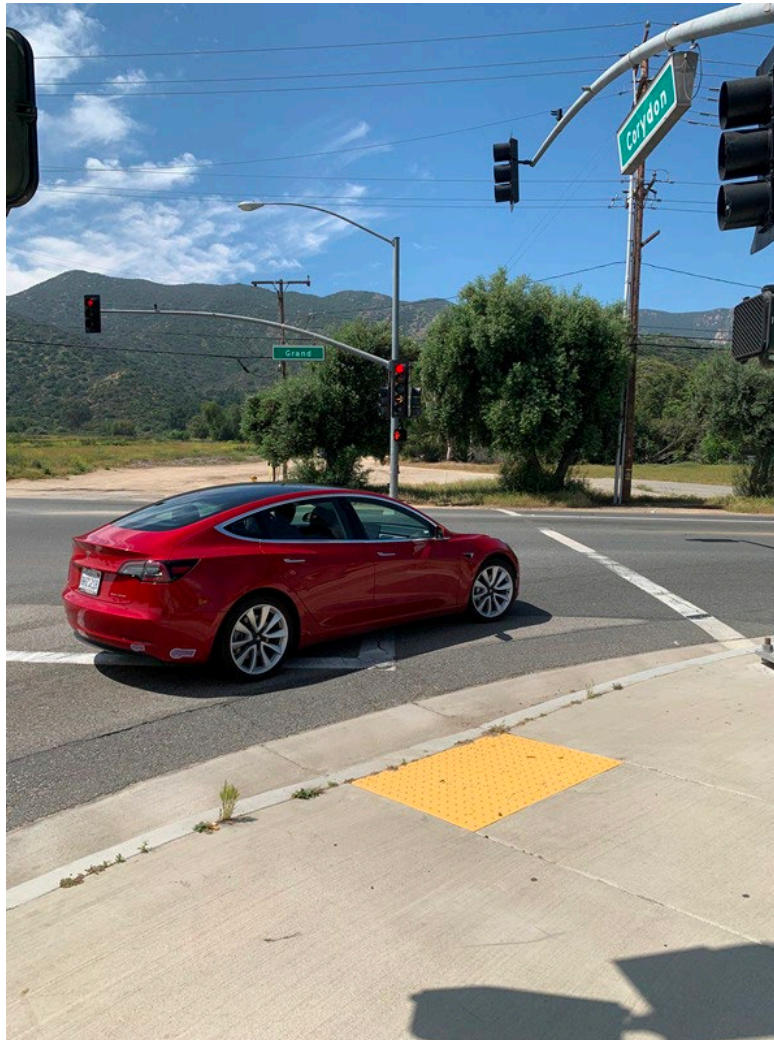
Figure 3.24: Street View of Southbound Corydon Road towards Grand Avenue
